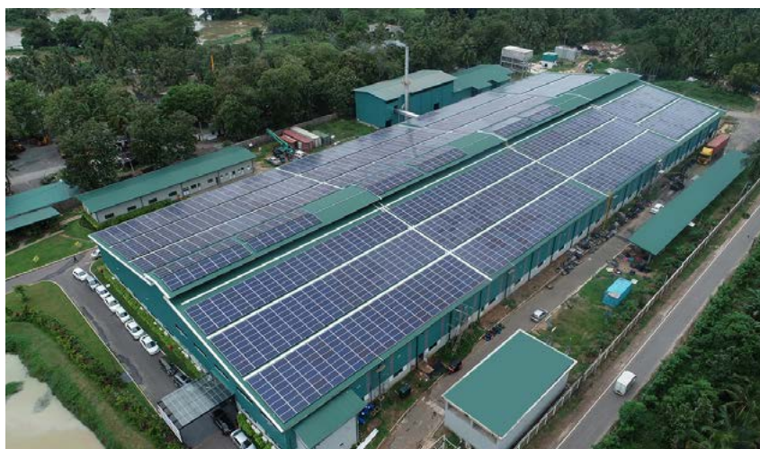
GRI Production Plant Expansion Progressing Well Despite Lockdown, image source: GRI Tires
