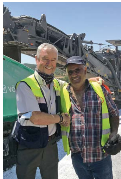
Foreman Pedro Silva from construction company Pragosa and Wirtgen recycling expert Mike Marshall (left) agreed that cold in-place recycling with the W 380 CR is extremely fast and economical. Image source: Wirtgen Group
