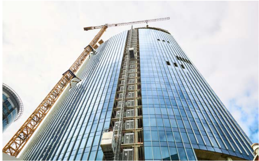
Skyscraper construction site in Brussels
